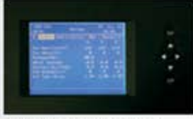
UPS Kabini Kontrol Paneli
